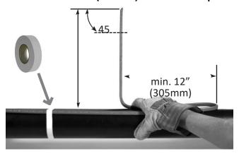
2. Push the cable up through the pipe stanchion piercing the grommet.
