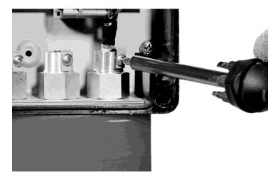
**13.** Install Core Sealer over bus wires.
