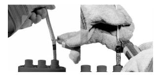
**9A.** Trim the braid back to the edge of the tape. **Do not damage the inner jacket.**
