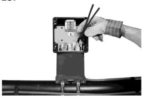
Feed field wiring power and ground conductors into the cutout in junction box using suitable wiring method. For hazardous location
