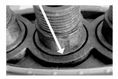
**3.** Feed cable(s) through the stanchion, piercing the grommet membrane.
