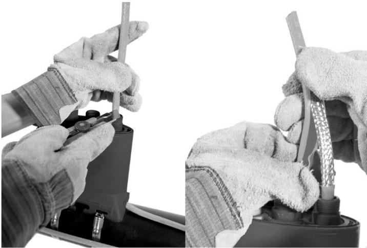
8. Wrap tape around the braid 1" (25 mm) from end of the outer jacket cut back.
