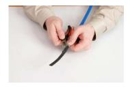
6. Cut down the middle of the inner core between bus wires. This can be done with a scissors or knife. The core sealer will fit over the bus wires while still encapsulated by the heater core. It is not necessary to expose the bare bus wires.
