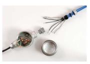
2. Twist Heater Cable Conductors together.
