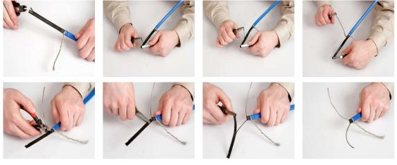
7. Place the supplied tube over one bus wire prior to sliding the core sealer over the bus wires (PGW, MT only - this will provide added protection from a short between the two bus wires). Then slide the core sealer over the bus wires of the cable, over the inner core until as close to the braid as possible.
